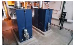
Typical wood pellet boilers
