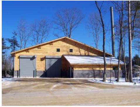
New wood chip storage and boiler facility at the Merrimack Valley High and Middle School
